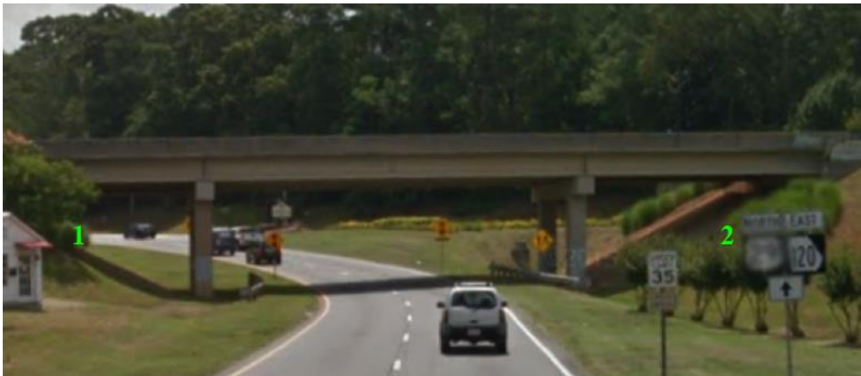
Figure B.5 Bridge 067-52520
