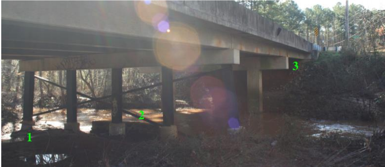
Figure B.6 Bridge 135-50880
