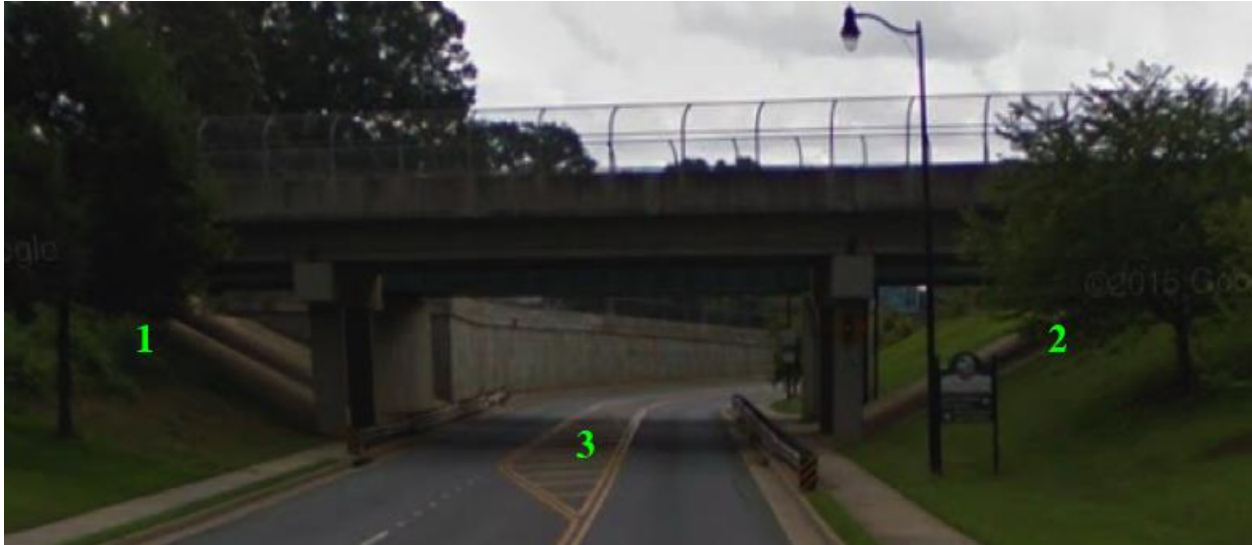
Figure B.4 Bridge 067-52520
